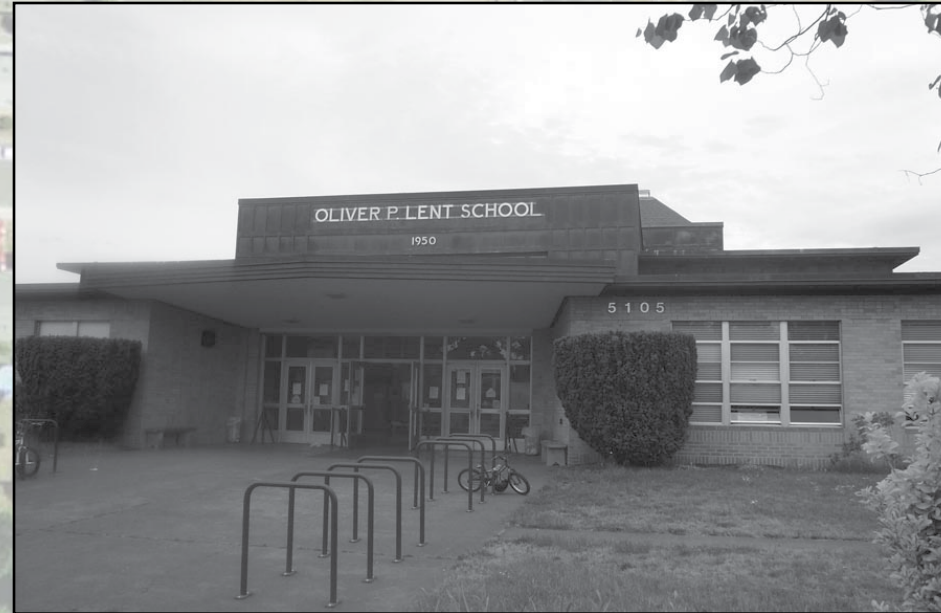
2009 photograph of the main entrance.
