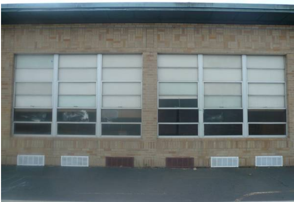
Brickwork facing north
