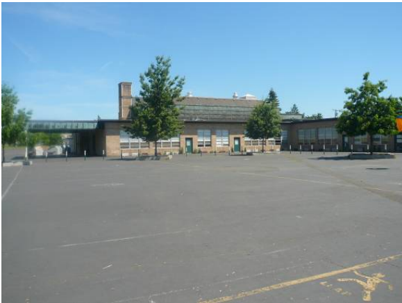
Southwest elevation facing northeast
