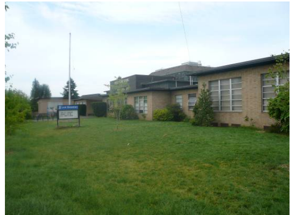
East elevation facing southwest
