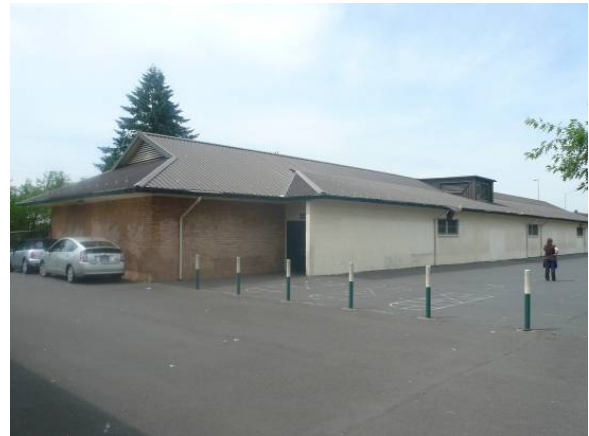
Addition facing southwest
