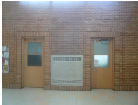
Corridor doors and brickwork
